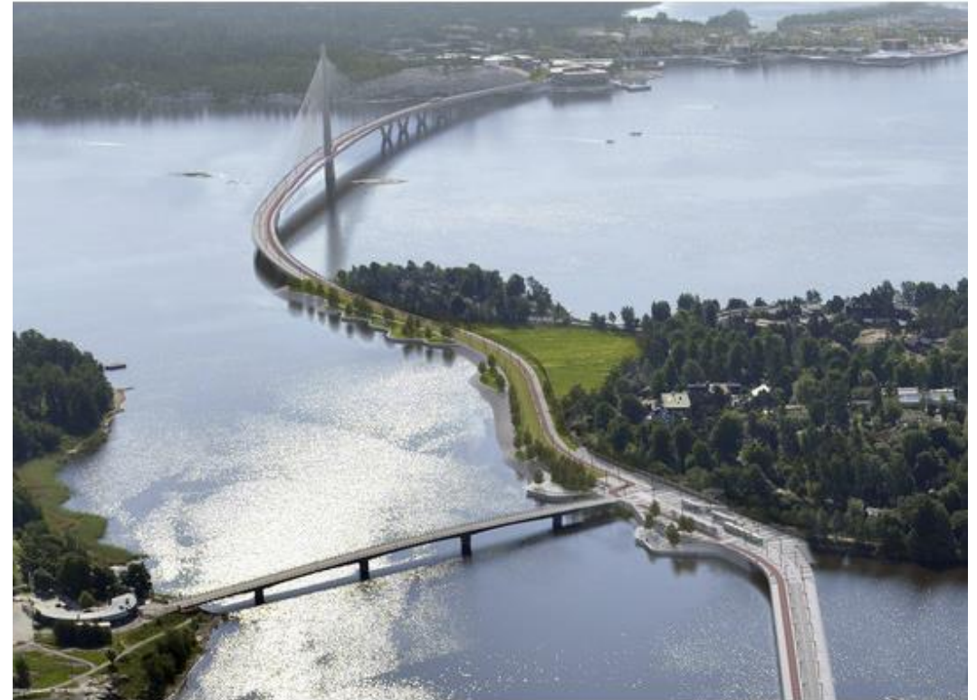
Rail and infra consulting services and structural engineering for a 10 km new light rail line connecting eastern and downtown Helsinki
